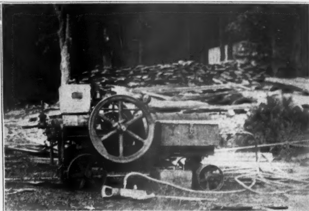
Portable Gasoline Engine Driven Compressor. Jackhammer Lying on Ground
